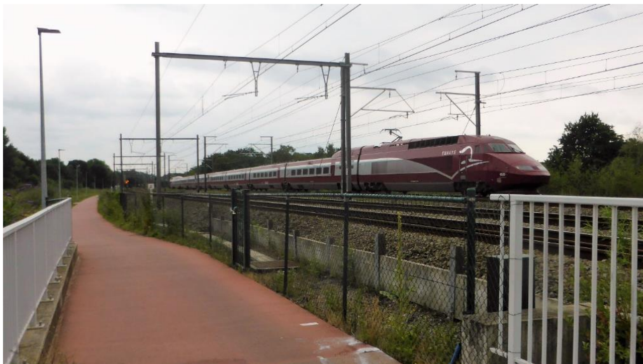
The F1 cycle highway in Belgium between Mechelen and Antwerp follows a high-speed TEN-T railroad line. The benefits of the investment exceed the costs by a factor of 14. 23 Photo credit: ECF.
